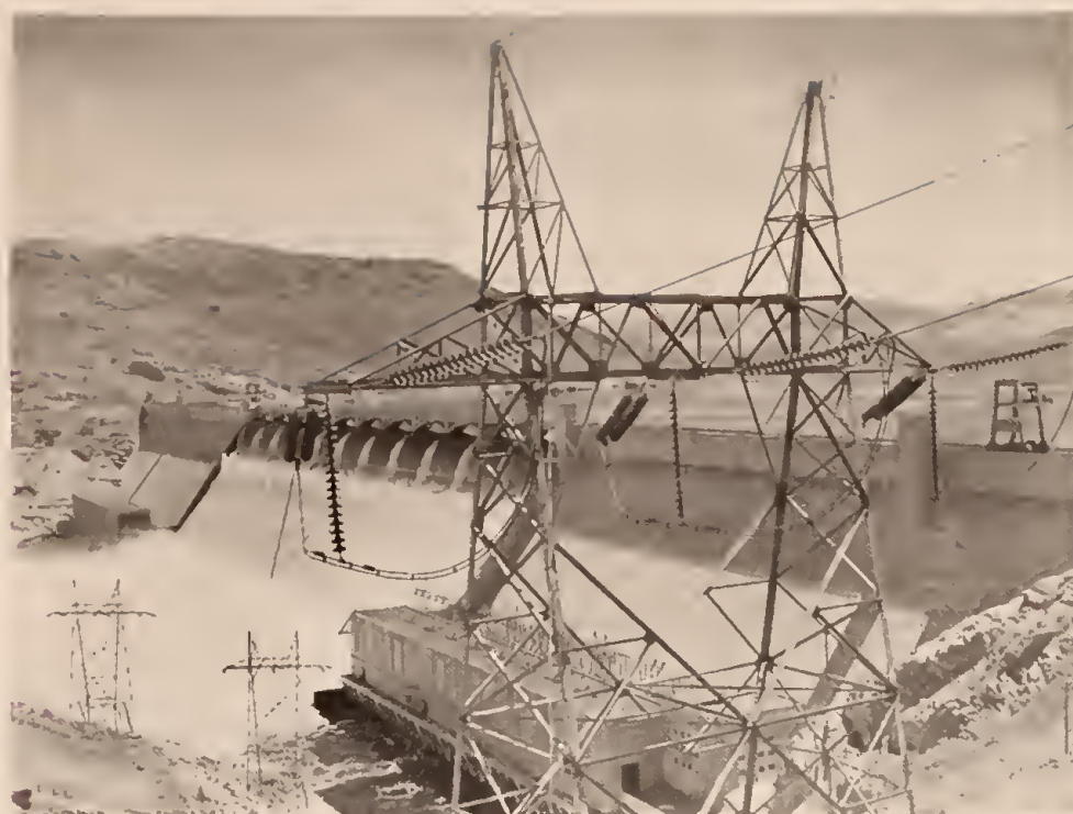
Federal engineers have been responsible for some of the world's greatest engineering projects. Career engineers have handled many mammoth projects from the blueprint stage through their completion and operation. Grand Coulee Dam is one of the huge multiple-purpose projects operated by the Government.
